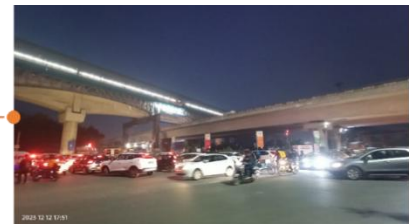
Absence of road markings, signages and speed control measures at the intersection.
