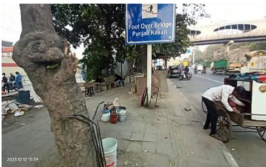
Obstructed pedestrian infrastructure
