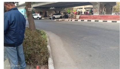
Absence of raised crossing for pedestrians at unsignalized junctions.
