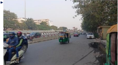
Absence of road markings, signages and speed control measures at the intersection.
