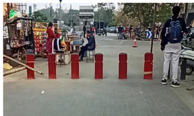
Inappropriate gap between bollards and absence of bollards at some places.
