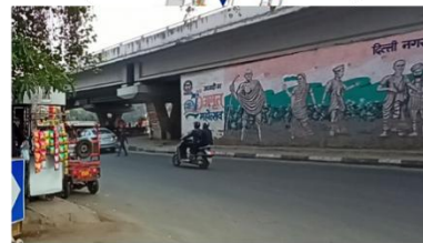
Absence of traffic calming measures like rumble strips near junctions.
