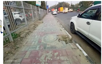
Absence of tactile flooring for differently abled users on outer ring road.
