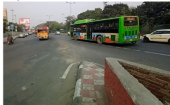
Absence of chevron marking.
