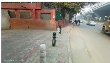
Absence of kerb ramps in front of crossing
