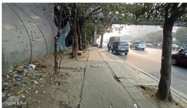
Damaged and obstructed pedestrian infrastructure
