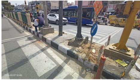
Obstructed refuse island
