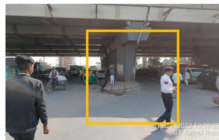
Haphazard parking at the bus bay, boarding & deboarding on the active main carriageway.
