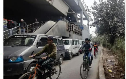
Pathway leading to subway is encroached by the car parking creating conflict for pedestrians and cyclists. Safety and security issues due to inadequate lighting.
