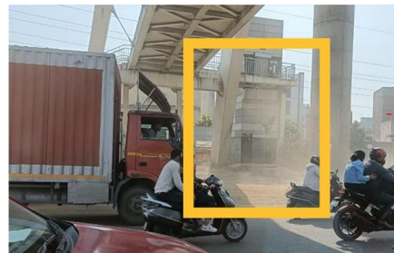
The lift is currently not functional, people do not take the foot over bridge and prefer to cross at-grade.
