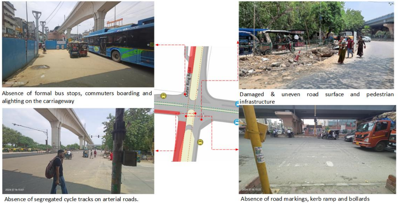
Figure 20: Issues identified at Peeragarhi Chowk
