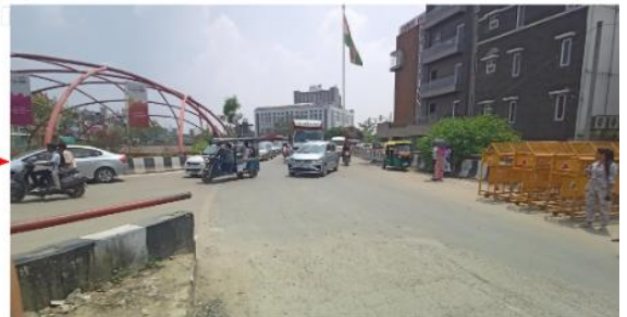
Absence of signages and speed control measures at the intersection.
