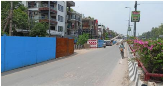
Absence of road markings
