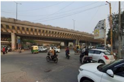
Absence of road markings, signages and speed control measures at the intersection.
