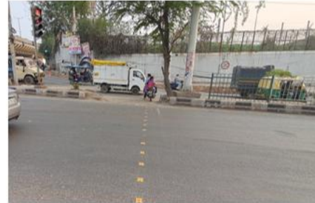
Absence of zebra crossing markings.
