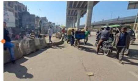
Absence of road markings, signages and speed control measures at the intersection.
