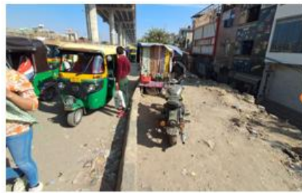
Damaged and obstructed pedestrian infrastructure on each arm.
