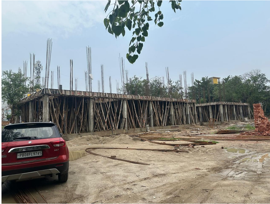
Figure 9 E-bus depot facilities under construction in Jalandhar
